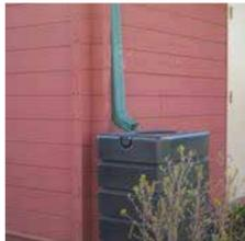
The Township already has installed a rain barrel on the main building in the Park. Rain barrels collect stormwater from downspouts and save it for later reuse. The water collected in the barrel can be used to water the other plantings in the Park.
