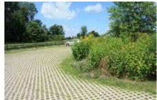
Porous paving allows water to move through the pavement and infiltrate back into the ground. This Best Management Practice could be installed in this high traffic area that appears to be used for car, tractor and golf cart parking.
