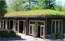
The six dugout roofs in the Park could be equipped with green roofs. A green roof is a roof that is covered in plants that absorb rainwater. There are various styles of green roofs that may be incorporated to show residents the feasibility of this BMP (Best Management Practice).
