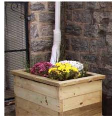
A downspout planter is a specially designed planter that connects to the roof downspout and stores, filters and uses rainwater. One or more of the downspouts from the main building could be connected to planters to show residents an easy and attractive stormwater BMP (Best Management Practice).
